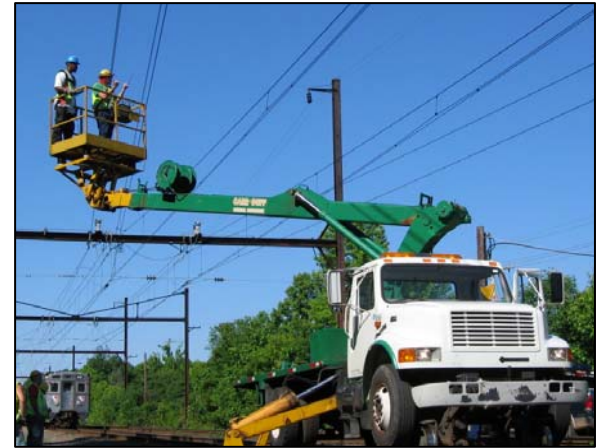
Catenary Replacement Doylestown Line
