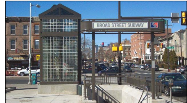
Allegheny Station ADA Improvements
