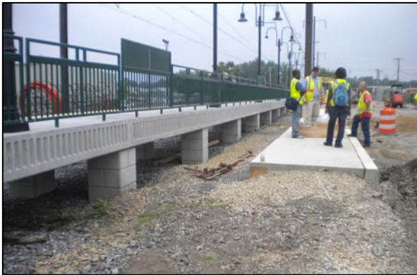
Primos Station Reconstruction
