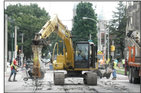
58 th and Chester Avenue Track Renewal Project
