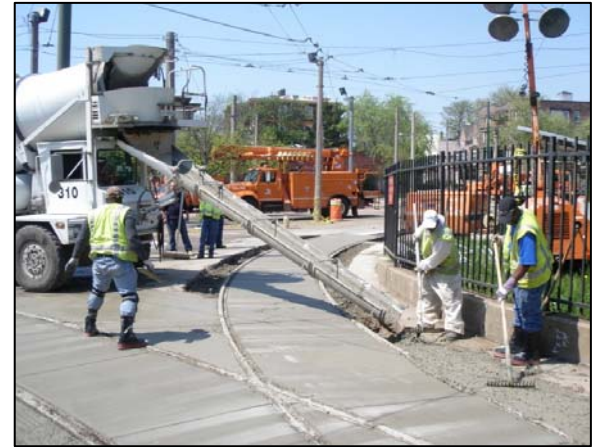
Special Trackwork Renewal 40th Street Trolley Portal
