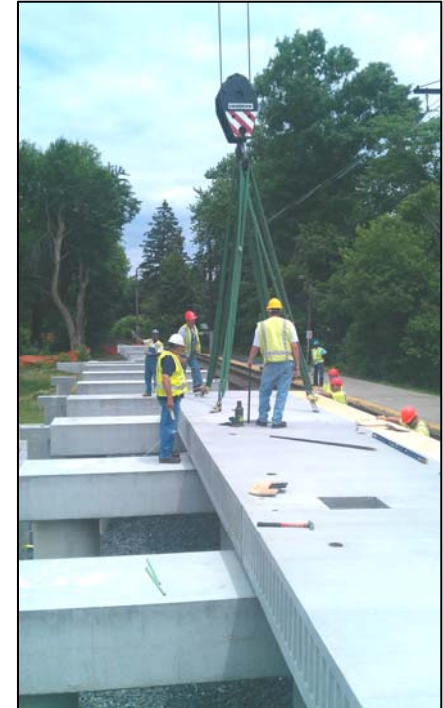
Ryers Station Reconstruction
