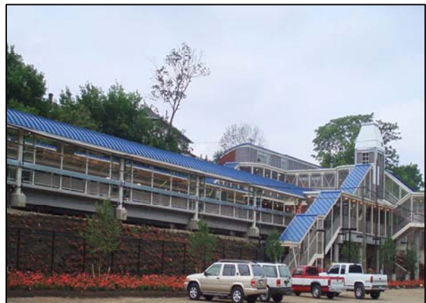
New Millbourne Station Entrance Area
