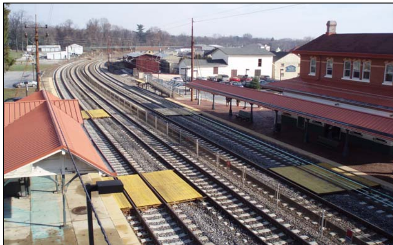
R5 Paoli Line Continuous Welded Rail and Concrete Crossties
