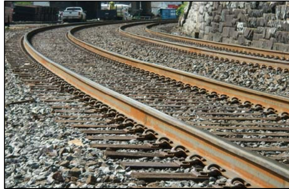
After – Continuous Welded Rail
