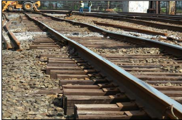
Before – Jointed Rail
