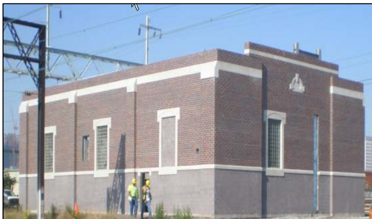
Construction of New Fairmount Substation
