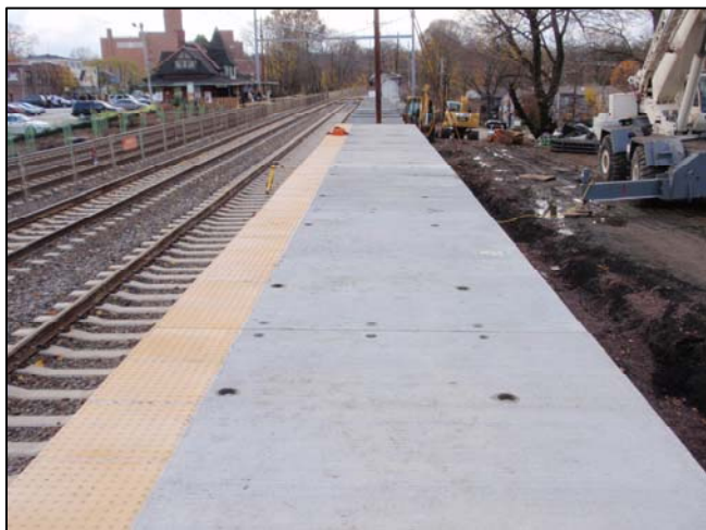
Wayne Station Improvements
