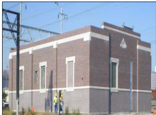
Construction of New Fairmount Substation
