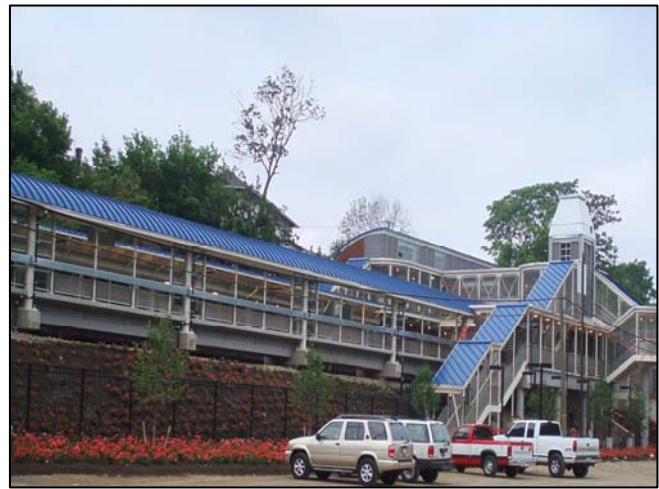
New Millbourne Station
